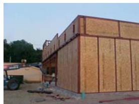
Exterior view of Superior Building.
